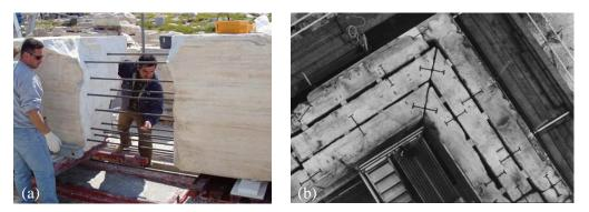
Figure 1: (a) In-situ restoration of one of the longest epistyles of the Acropolis Propylaea using threaded titanium bars; (b) Inter-connecting epistyles of the Parthenon Temple using "I"-shaped titanium beams.
